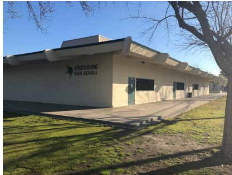
Exterior of Building 10 (rooms 10-15)
