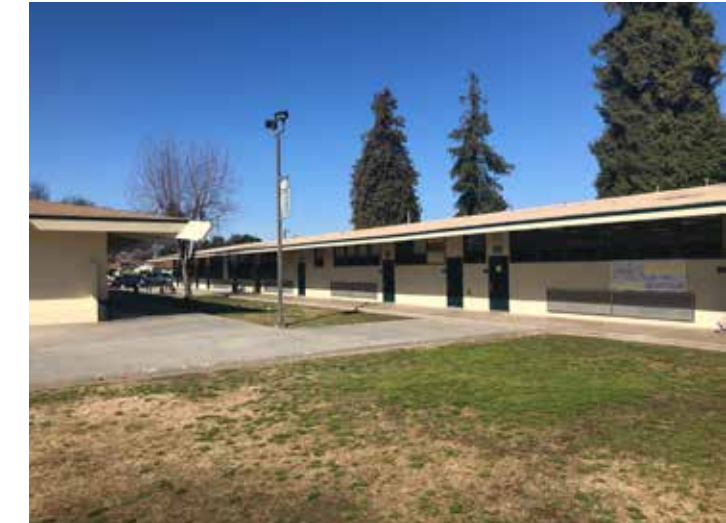
South side of Building 40
