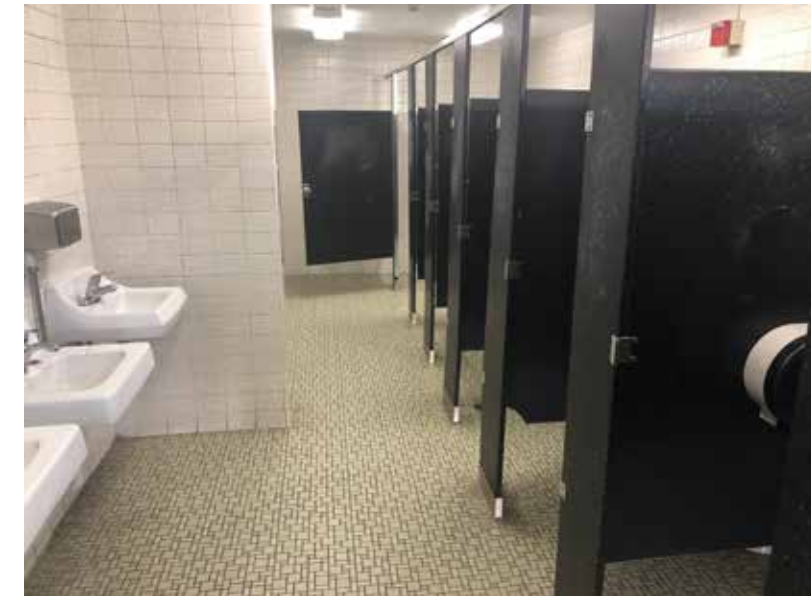
Non-compliant ADA restroom
