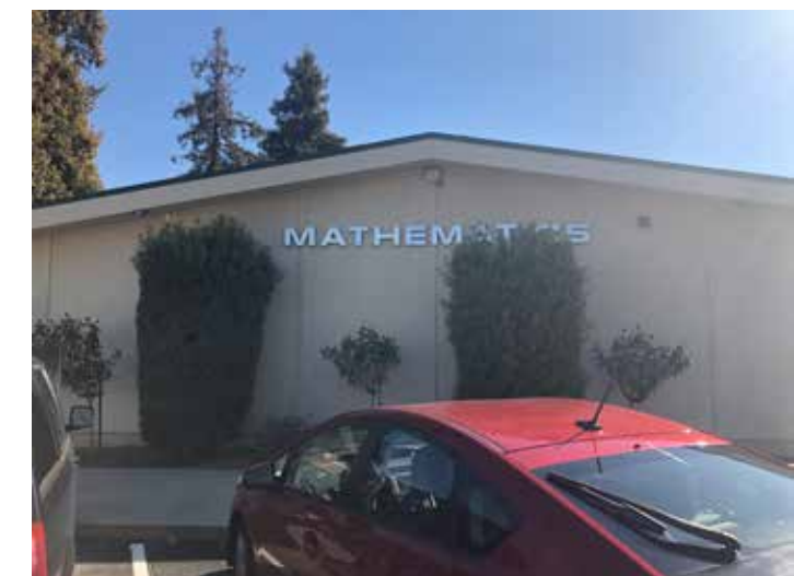
West end of Building 40
