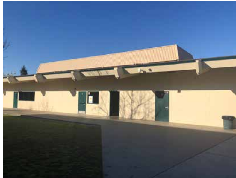
Exterior of Building 80 (rooms 80-87)
