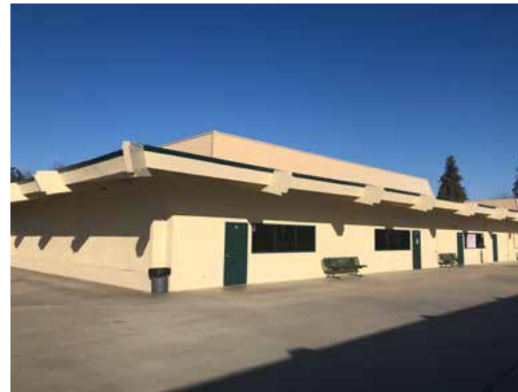
Exterior of Building 20
