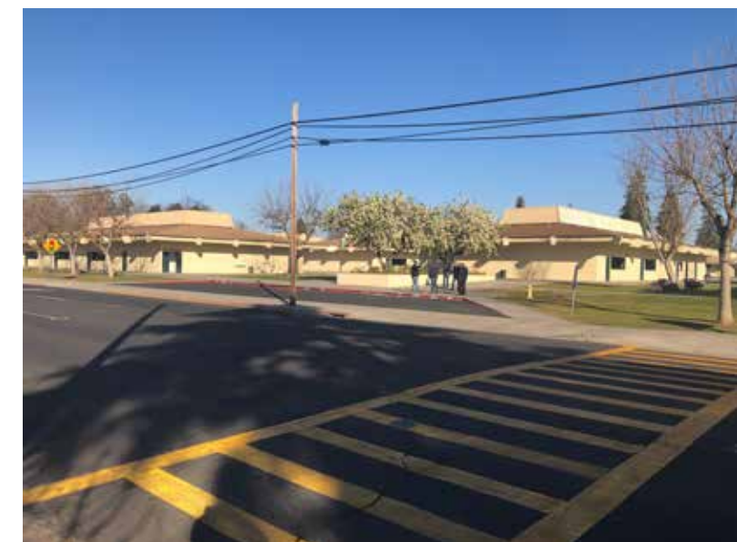
Exterior of Building 80 (rooms 80-87)
