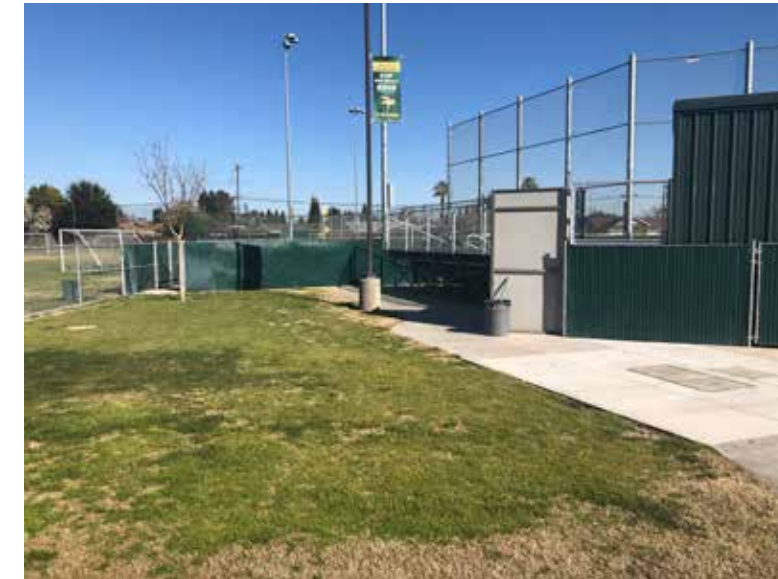
Softball field access lift
